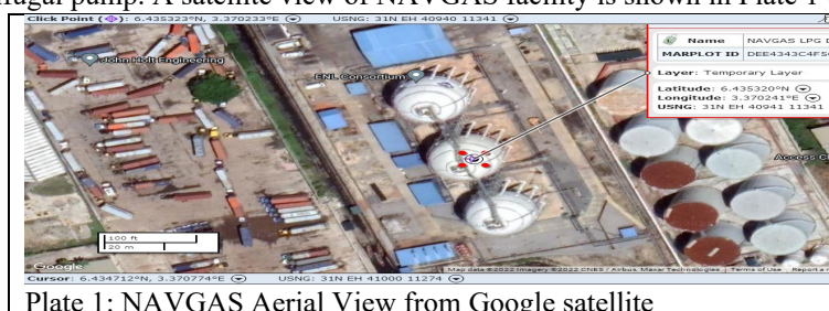
Plate 1: NAVGAS Aerial View from Google satellite
